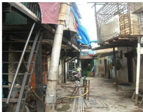
Illegal water connections
